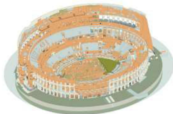
Figure 17: Digital HBIM reconstruction of the Colosseum from point clouds, enabling detailed documentation and heritage management.
