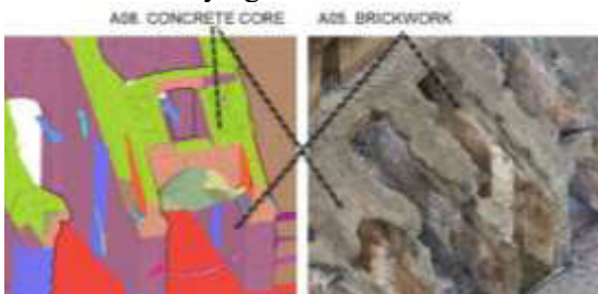
Figure 13: 3D mapping of opus testaceum, distinguishing the concrete core from the brickwork.
